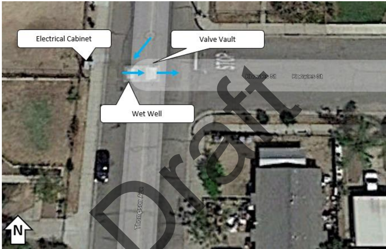
Figure 7-8 Aerial View of Sunset Lift Station
