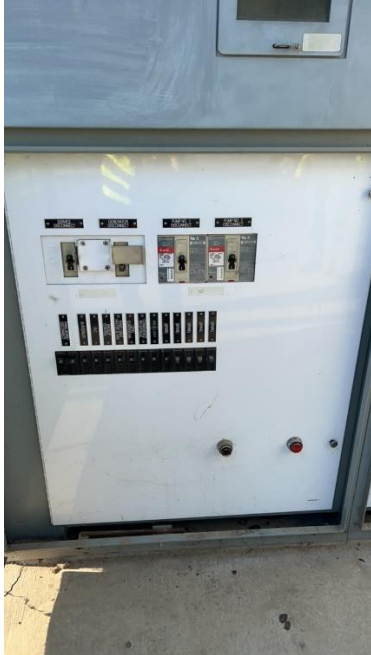
Photo 7-33 Electrical & Power – Meter/main section replaced in 2005
