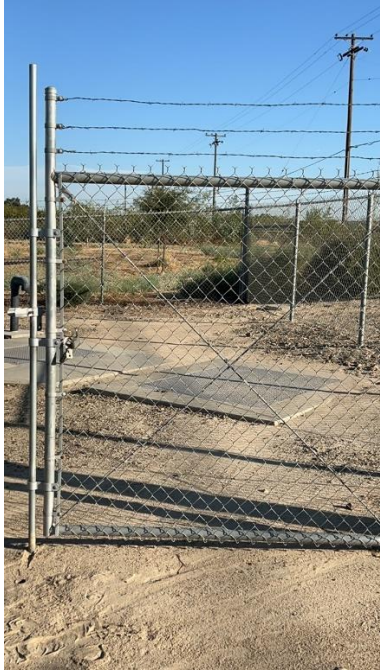
Photo 7-25 Site / Civil – Chain link fence in good condition
