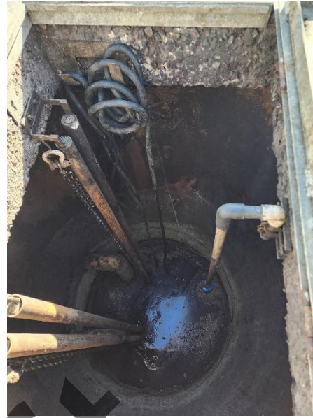
Photo 7-30 Site / Civil – Wet well from original plant
